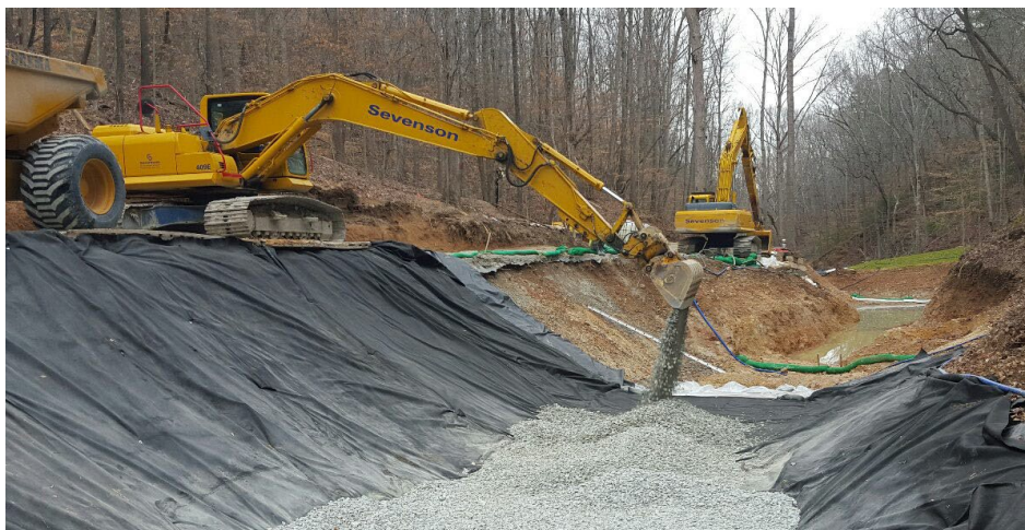
Surface Water Flow Being Rerouted Around the Work Area
