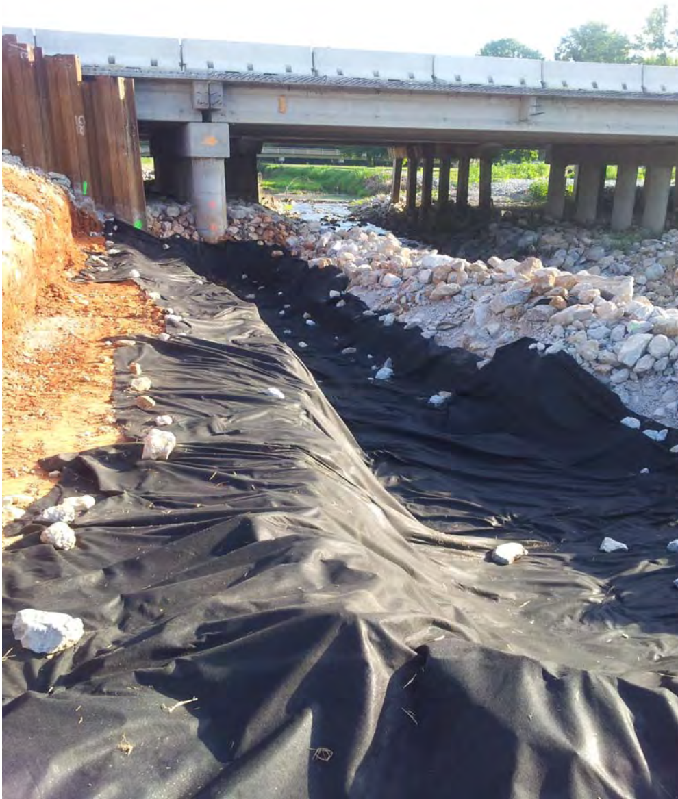
Photo 11: Geotextile installation at Bent 2. Photo looks north.
