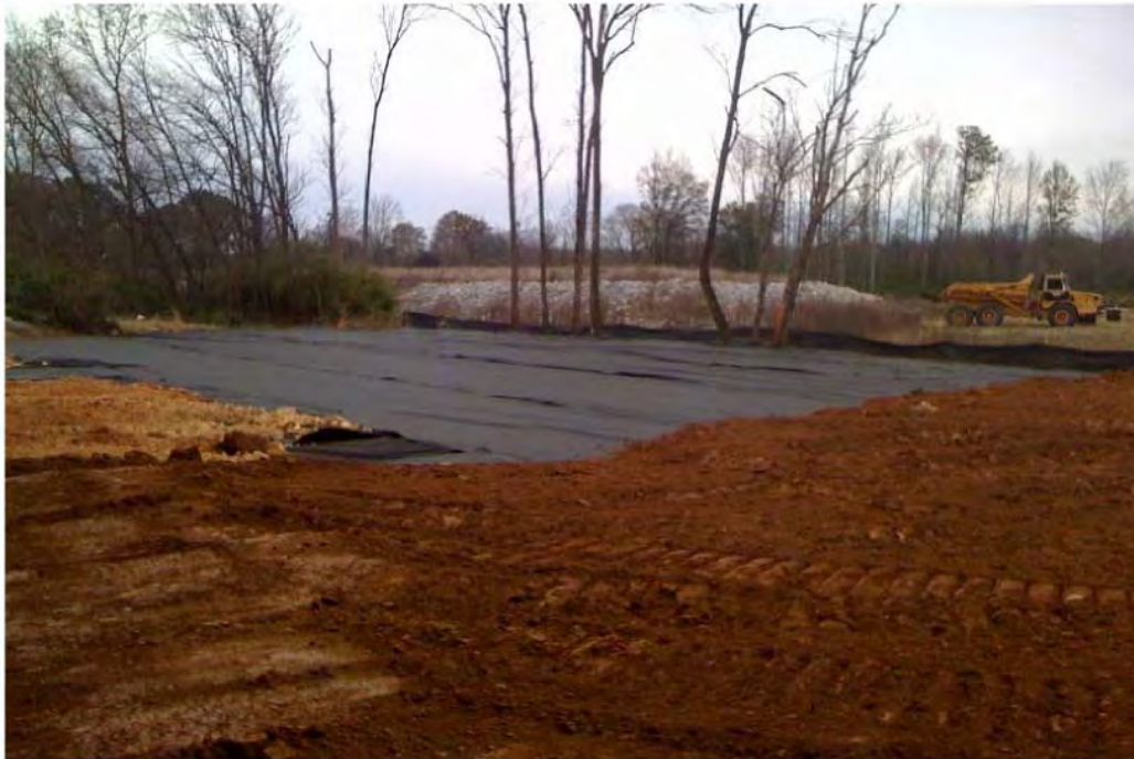
Photo 3: Geotextile marker layer and clean cover installation in Bridge Area. Photo looks southeast.
