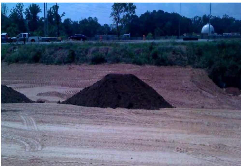
Photo 8: Clean cover installation in Northwest Quadrant. Photo looks southwest.
