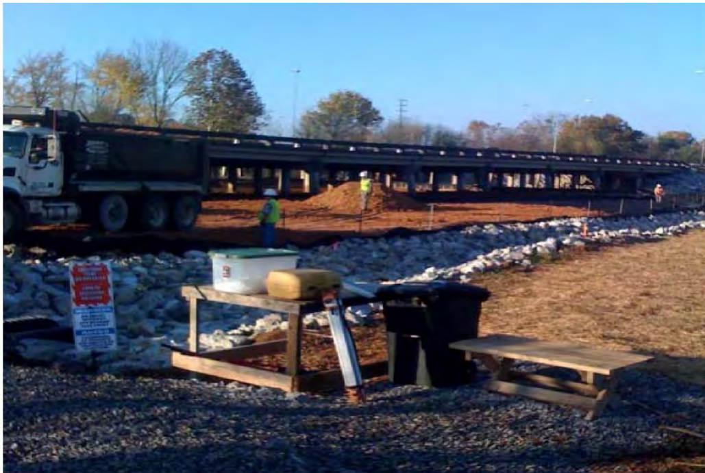
Photo 1: Bridge Area grading and clean cover installation with completed Northeast Ditch in foreground. Photo looks southwest.
