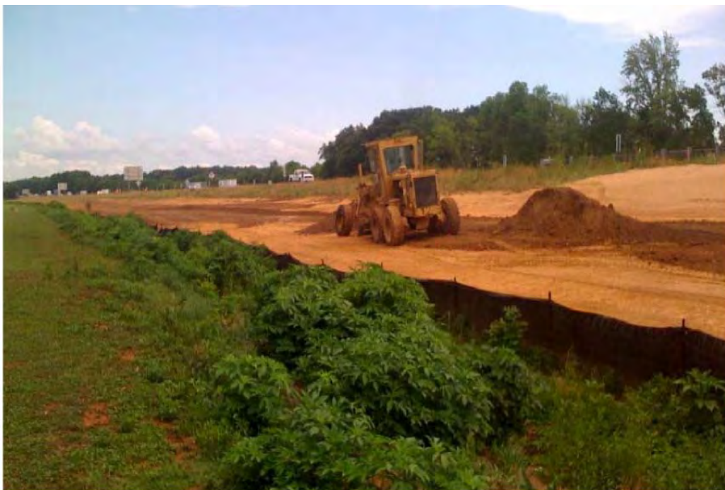
Photo 7: Clean cover installation in Northeast Quadrant. Photo looks southeast.
