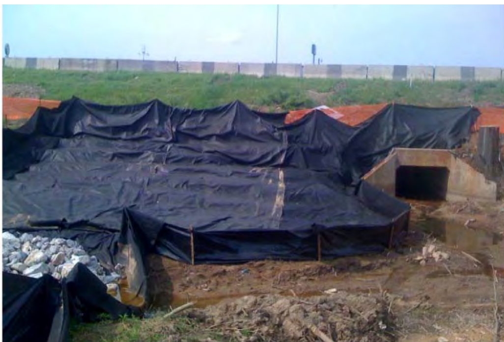
Photo 6: Southwest Quadrant soil embankment geotextile marker layer prior to clean fill cover. Concrete box culvert is shown to the right in photo. Photo looks north.
