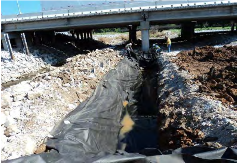
Photo 12: Bent 3 geotextile installation. Photo looks north.
