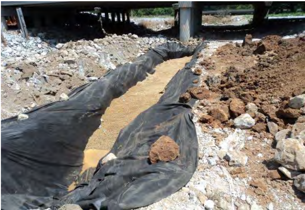
Photo 13: Bent 3 aggregate installation. Photo looks north.
