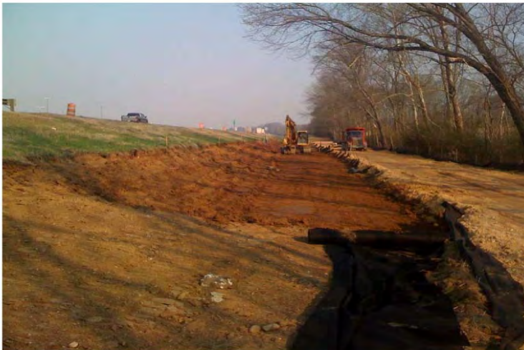
Photo 4: Soil Embankment and Floodplain grading/preparation for clean cover installation in Southeast Quadrant. Photo looks east.
