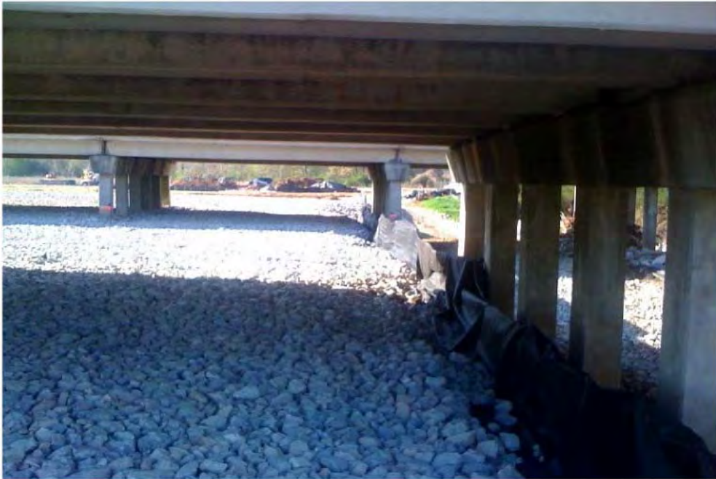
Photo 14: Six-inch gravel layer installed on top of clean soil cover in Bridge Area. Photo looks south.
