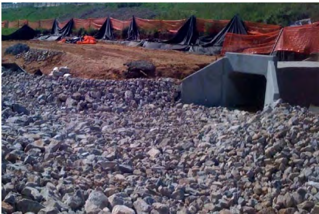
Photo 18: Southwest Quadrant concrete Box Culvert extension and new headwall and Southwest Ditch. Photo looks northwest.
