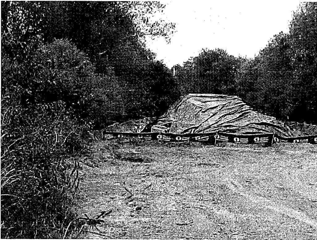
Photo 5: Phase I – Peak Flow Pump Station covered soil stockpile area with silt fence barrier.
