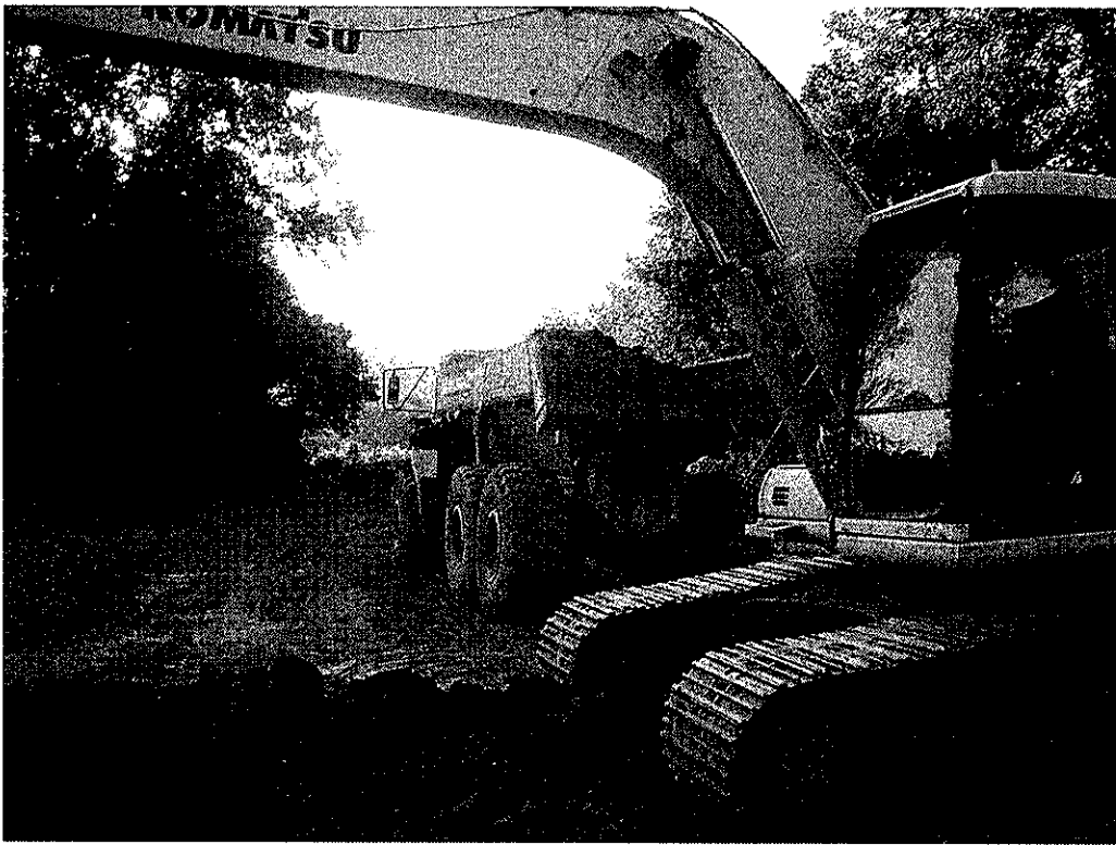
Photo 17: Phase II – Excavation and loading of impacted soils from Stormwater piping trench.
