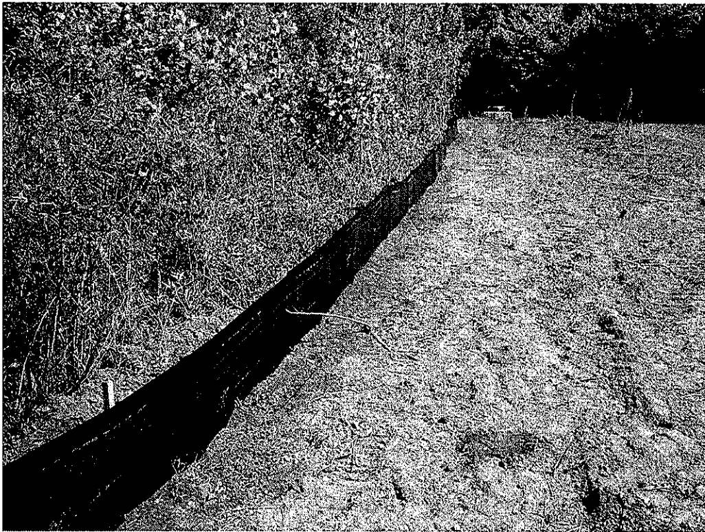
Photo 9: Phase II – Silt fence installation in Deep Bed Filter Units area.
