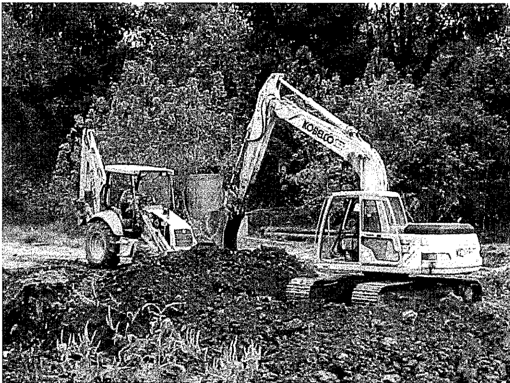
Photo 4: Phase I – Excavation and loading of soils from Peak Flow Pump Station area.
