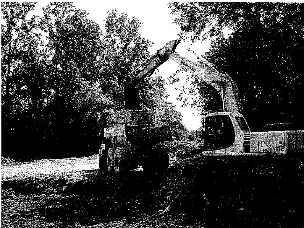
Photo 18: Phase II – Excavation and loading of impacted soils from flume area.
