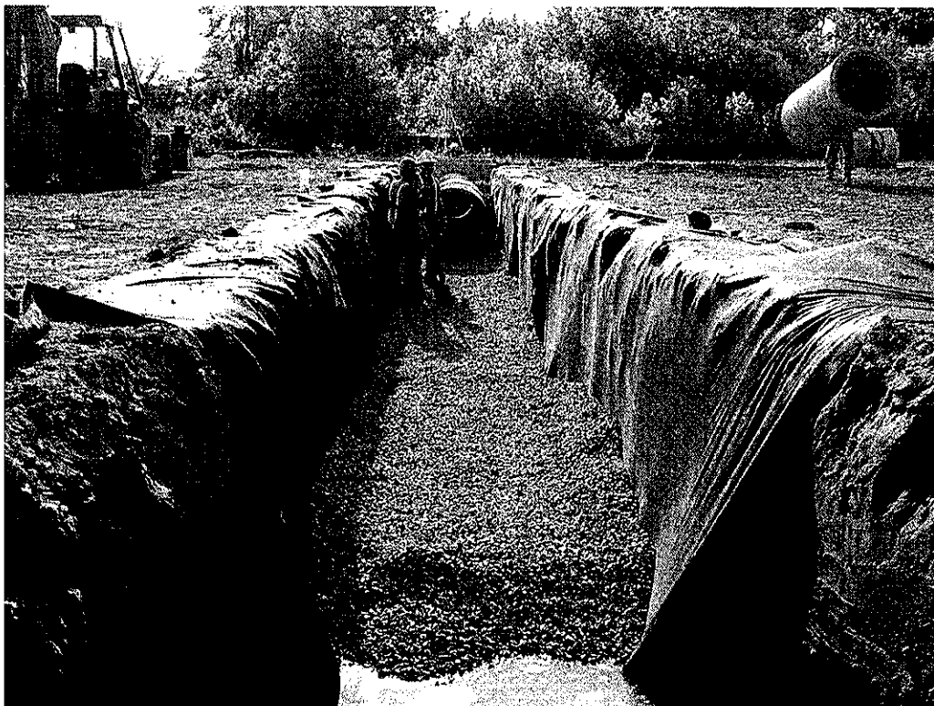
Photo 15: Phase II – Stormwater piping installation.
