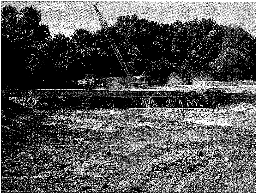
Photo 10: Phase II – Excavation and loading of impacted soils from Deep Bed Filter Units area.
