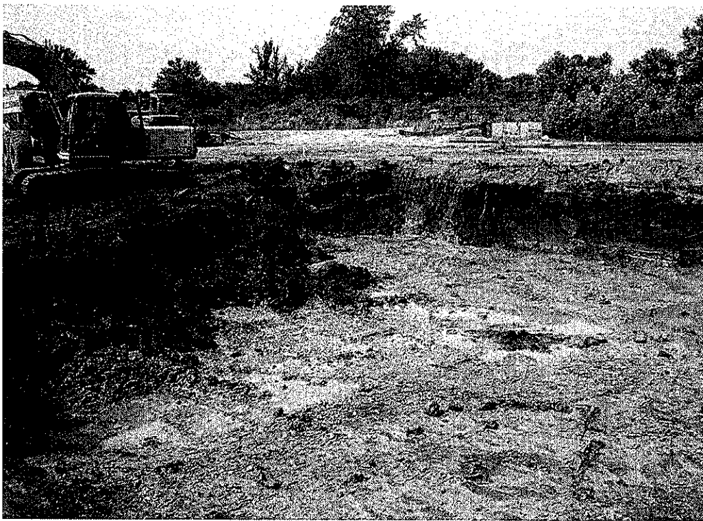
Photo 11: Phase II – Excavation and loading of impacted soils from Deep Bed Filter Units area.
