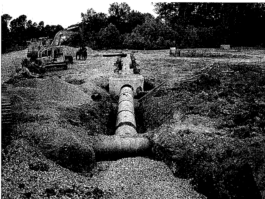
Photo 16: Phase II – Stormwater piping installation.
