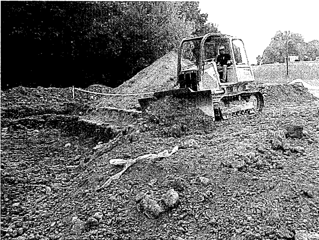
Photo 6: Phase I – Peak Flow Pump Station area clean fill cover installation.
